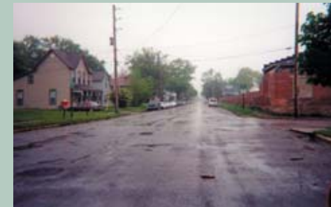
② View south along Plum Street
